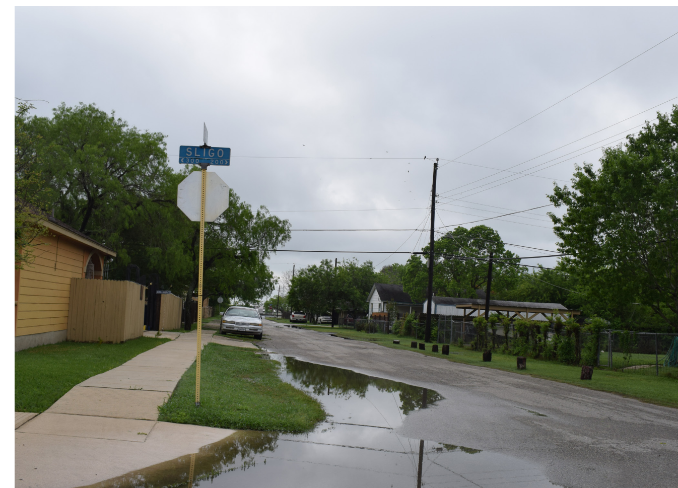
Poor drainage in the Brookside neighborhood
