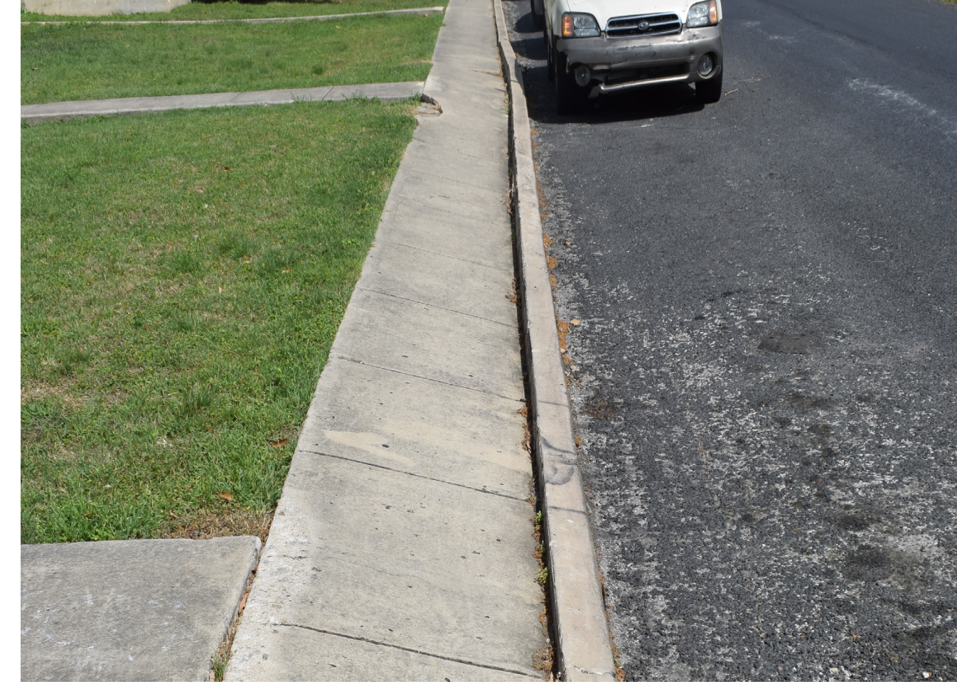
Poor sidewalk conditions in Highland Hills
